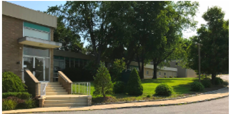
The new home for Cardinal Kung Academy
